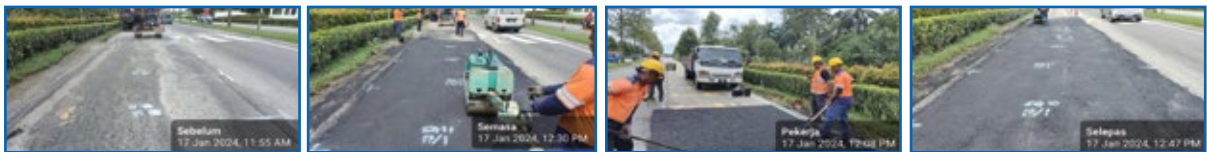
Jalan Senai Airport City
